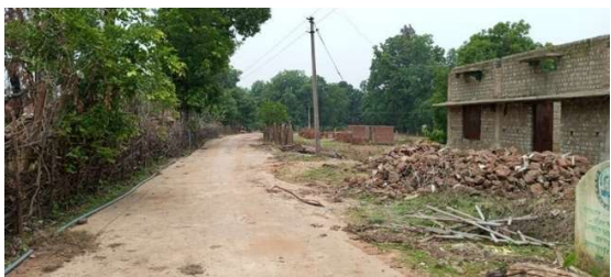
This Samudayik bhawan in Village Mhuahar, Panchayat Kerakachhar is delayed
