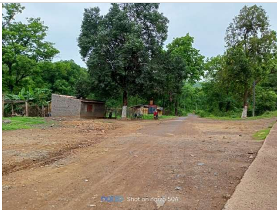
Construction of Jamudihi Road to Barsuan road, Gaganaposh of Chordhara Panchayat (Koida). It has damaged fast and requires attention.
